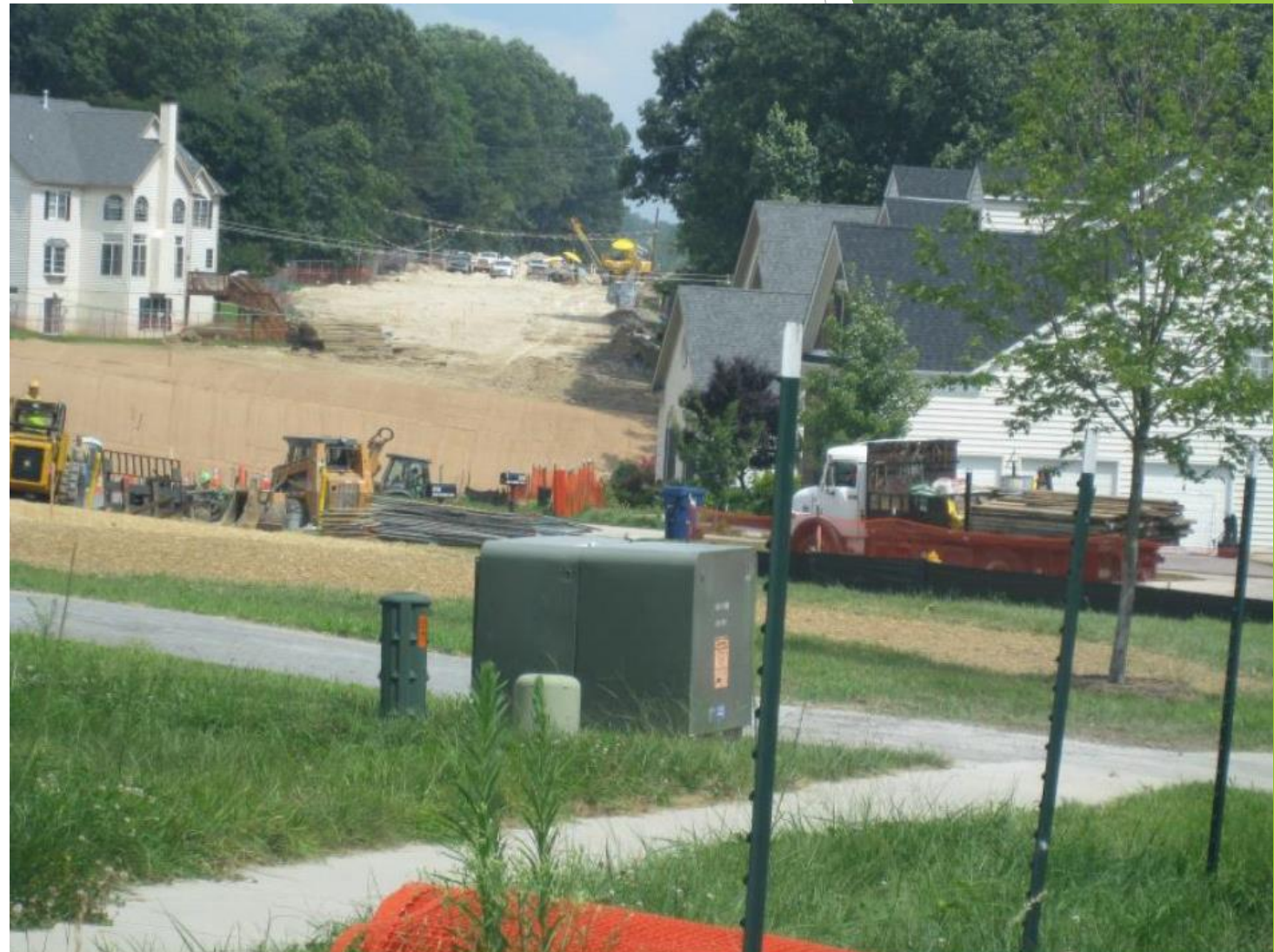
Chester County Residential Pipeline Worksite 2008
