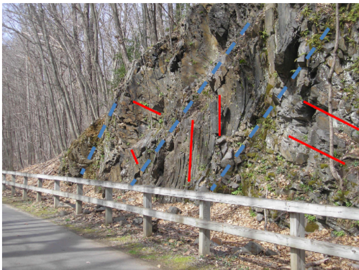
Photo 2: Note the rock orientation lines in RED and the Fault Lines in Blue Dashes .
